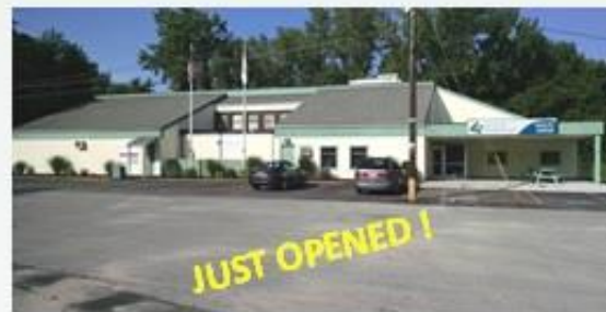
33 Maple Avenue North Providence
